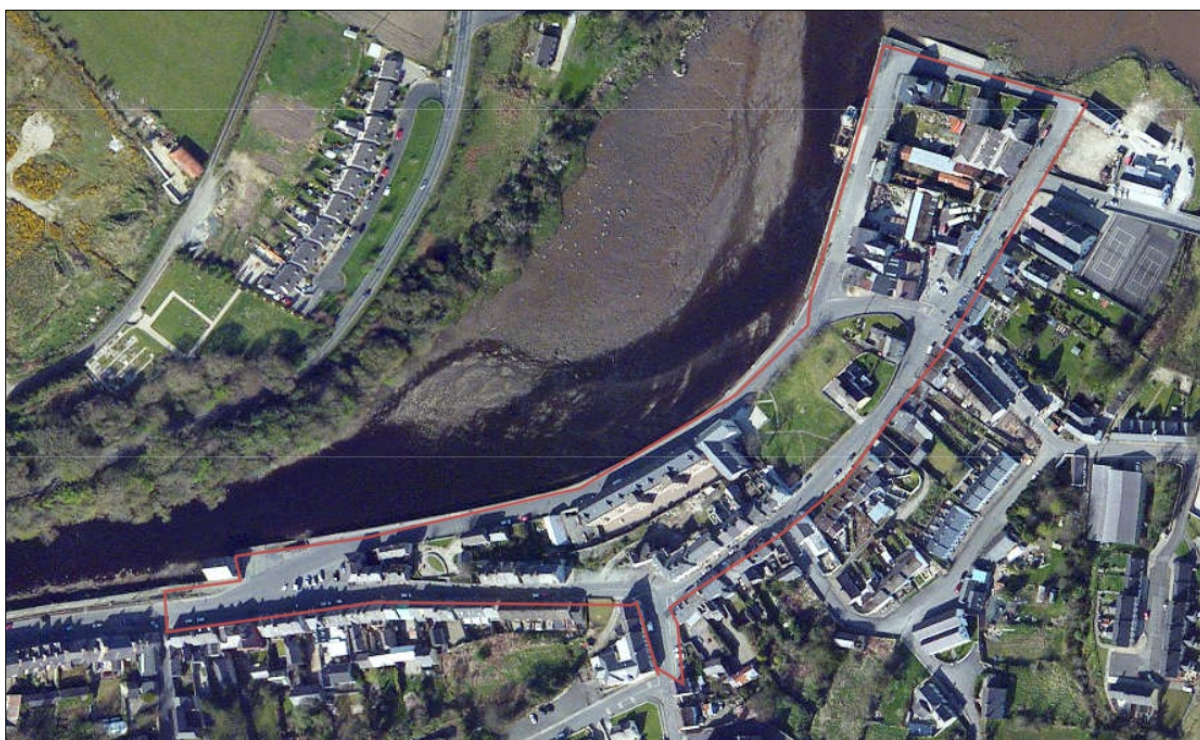
Figure 2: Aerial image of the Ramelton with public realm scheme boundary in red
