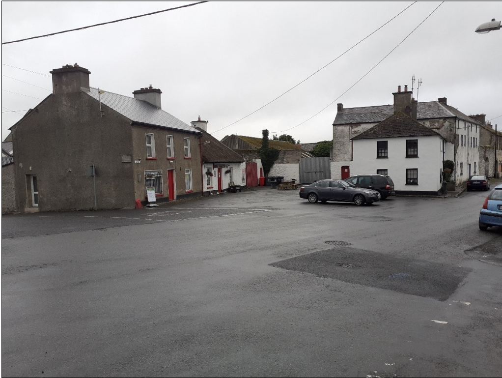
Plate 3: Public realm project area 'Market Square' facing northwest from the junction of Castle Street and Pound Street
