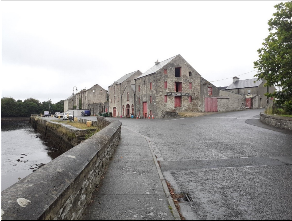
Plate 1: Public realm project area 'The Quays' facing northeast
